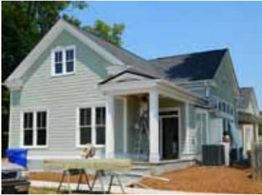
Painters put finishing touches on Charles House-Winmore
