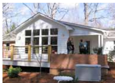
Back deck, Charles House-Yorktown
